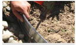
Drive spikes through holes in edging at a 45 degree angle. Start with the beginning piece of edging.
