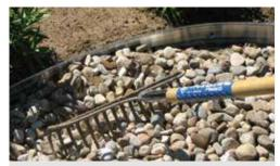
Stake and backfill edging continuously to ensure straight lines, compacting both sides to ensure the finish grade is approximately 1/2" below top of edging.
